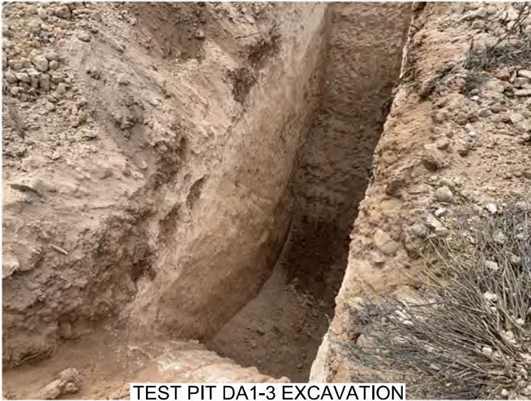
TEST PIT DA1-3 EXCAVATION
