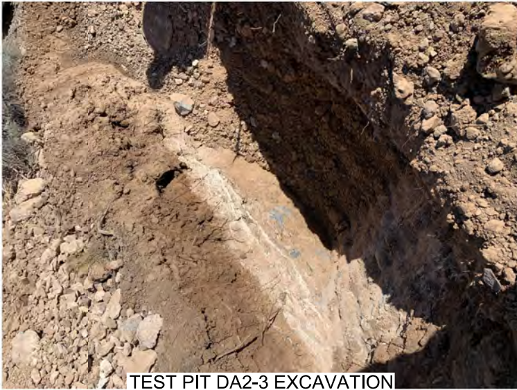
TEST PIT DA2-3 EXCAVATION
