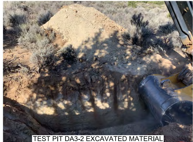
TEST PIT DA3-2 EXCAVATION
