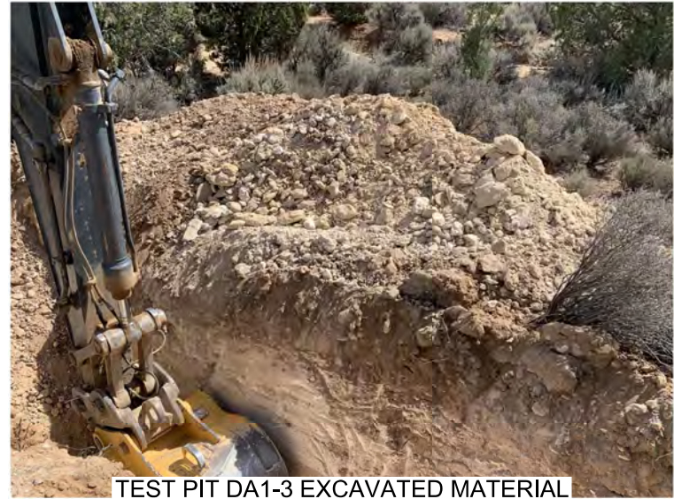
TEST PIT DA1-3 EXCAVATED MATERIAL
