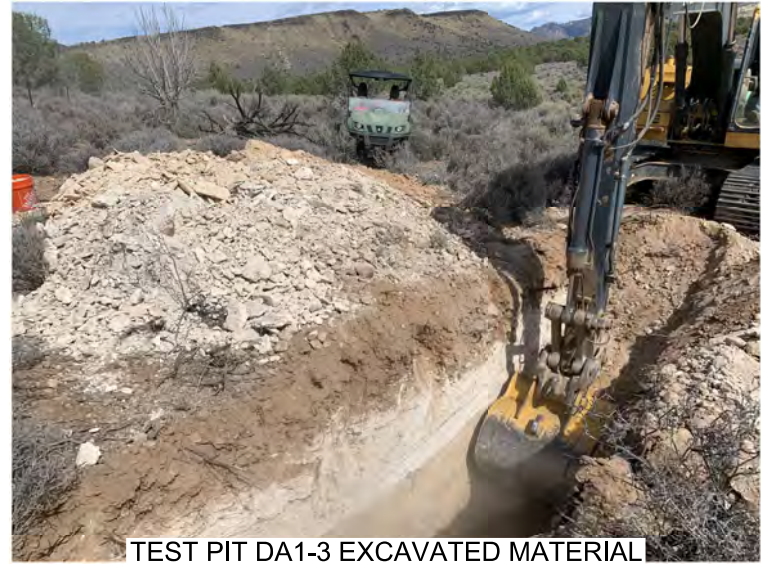
TEST PIT DA1-3 EXCAVATED MATERIAL
