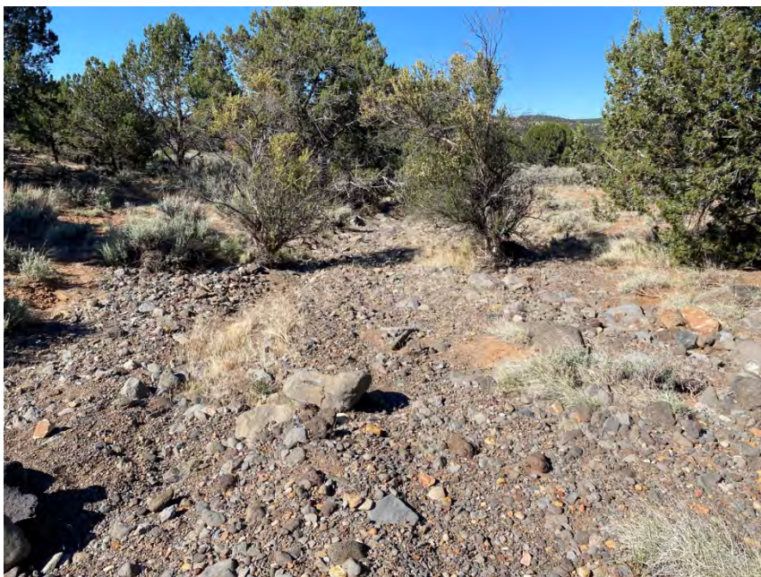
View of Wash 5 looking downstream where it exits the review area (facing west)
