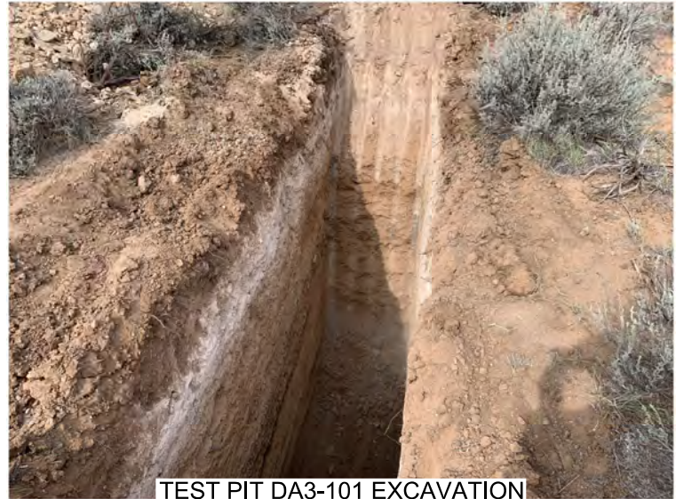
TEST PIT DA3-101 EXCAVATION
