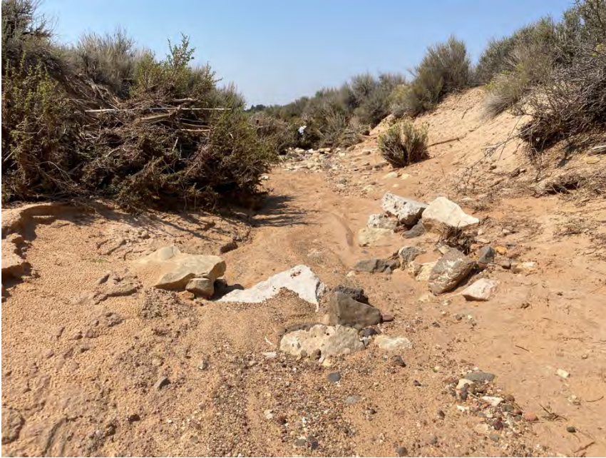
View of Wash 4 looking downstream where it enters the review area (facing west)
