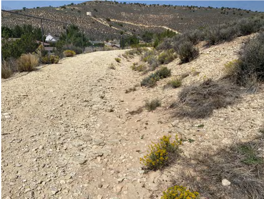
View of Wash 8 looking downstream (facing north)
