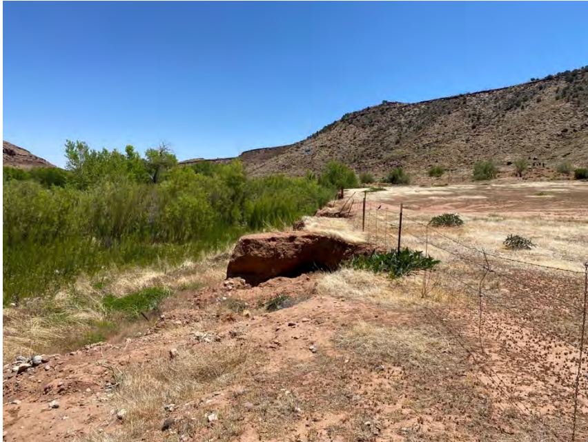
View of heavily eroding upland area adjacent to the Santa Clara River (facing east)
