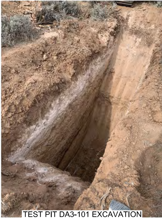
TEST PIT DA3-101 EXCAVATION
