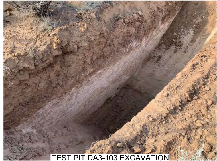
TEST PIT DA3-103 EXCAVATION
