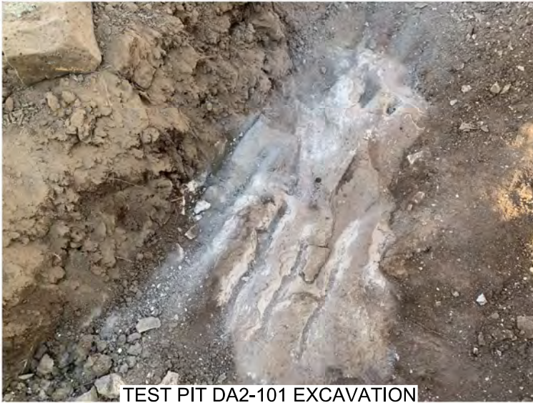
TEST PIT DA2-101 EXCAVATION
