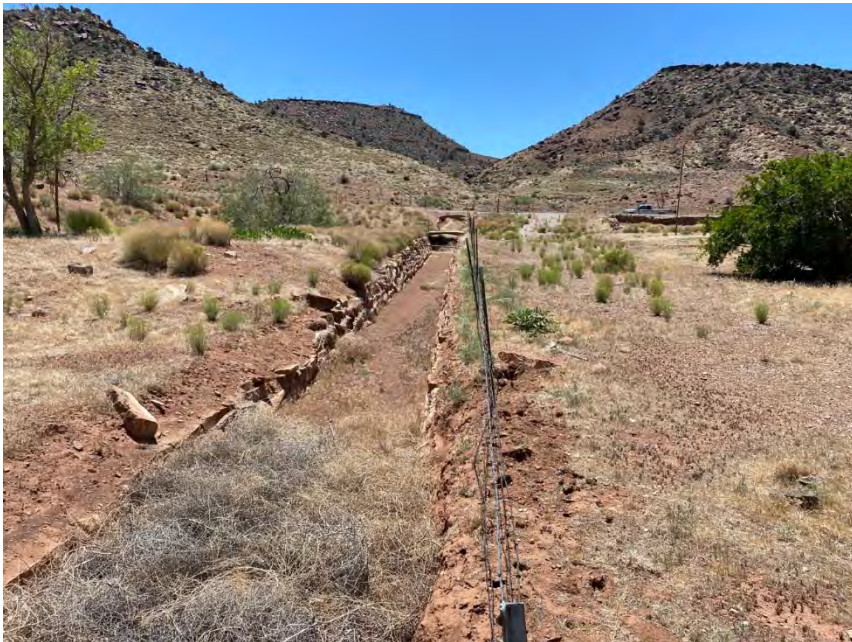
View of the improved section of Ditch 2 looking upstream (facing southwest)
