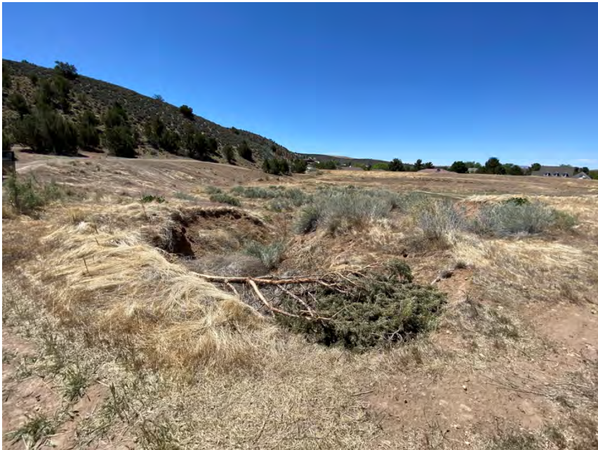
View of detention basin in northwestern corner of the southern section of the Dammeron Valley Review Area (facing southwest)
