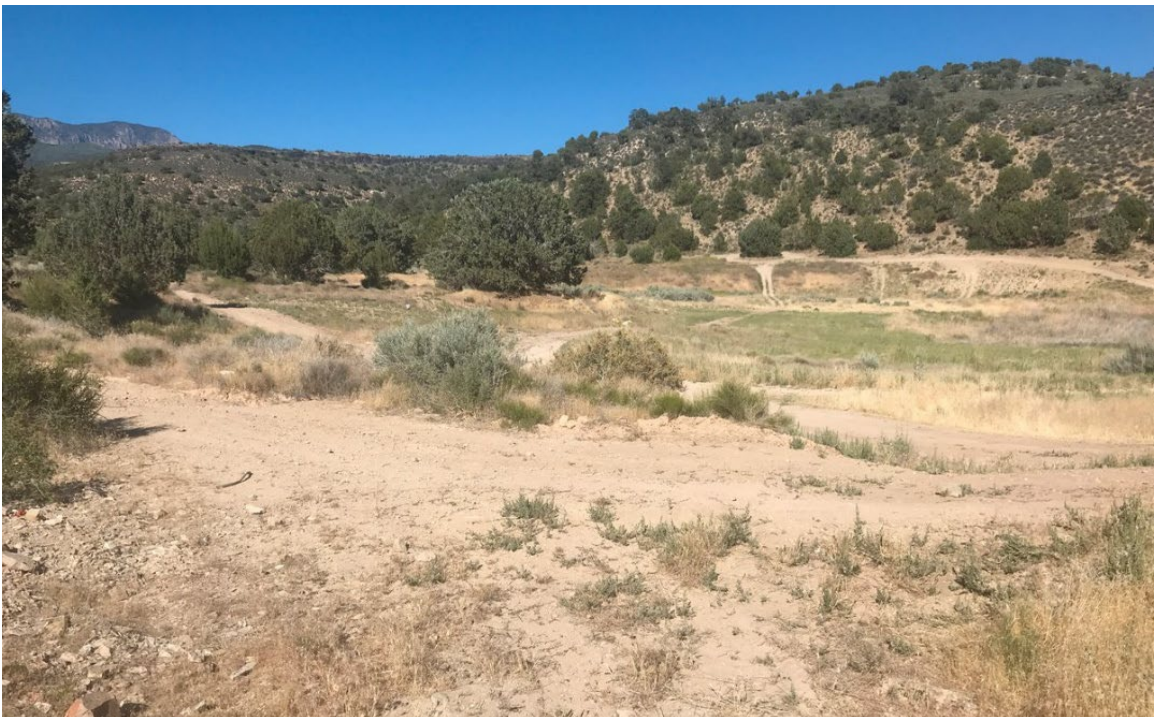
Photograph C-15. Existing Basin in Diamond Valley that would be repaired.
