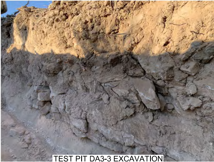
TEST PIT DA3-3 EXCAVATION
