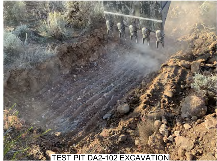
TEST PIT DA2-102 EXCAVATION
