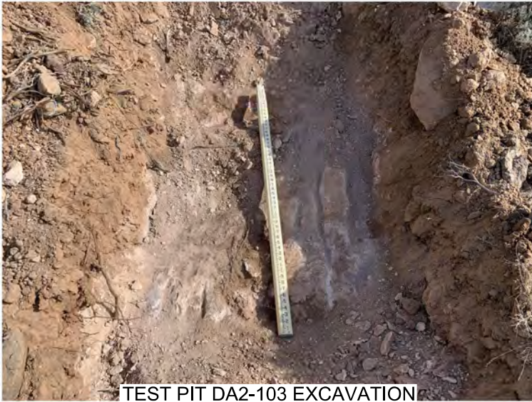
TEST PIT DA2-103 EXCAVATION
