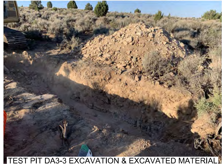
TEST PIT DA3-3 EXCAVATION & EXCAVATED MATERIAL
