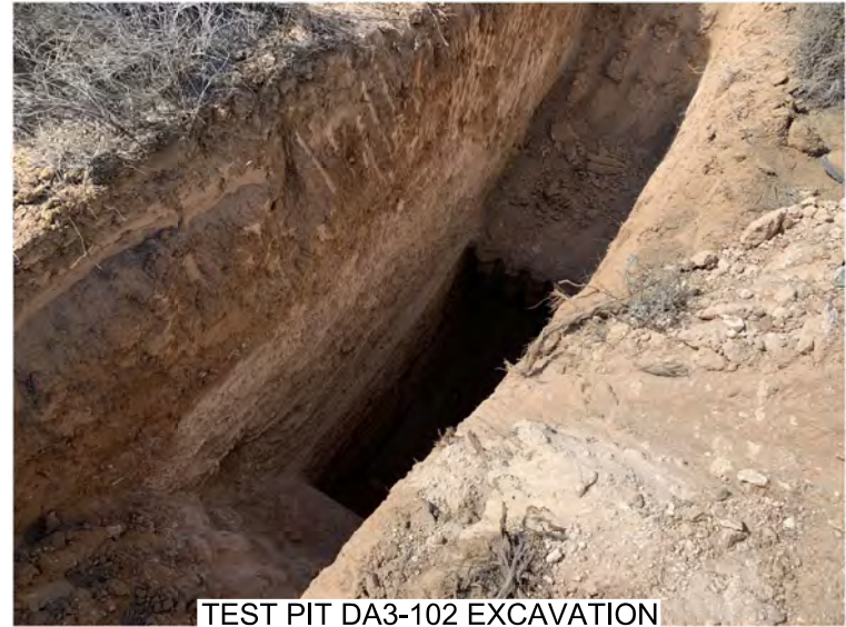
TEST PIT DA3-102 EXCAVATION
