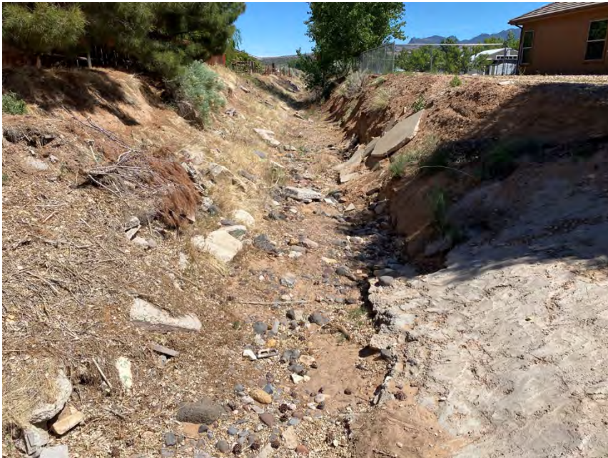
View of Wash 6 looking upstream from W Jade Dr (facing north)
