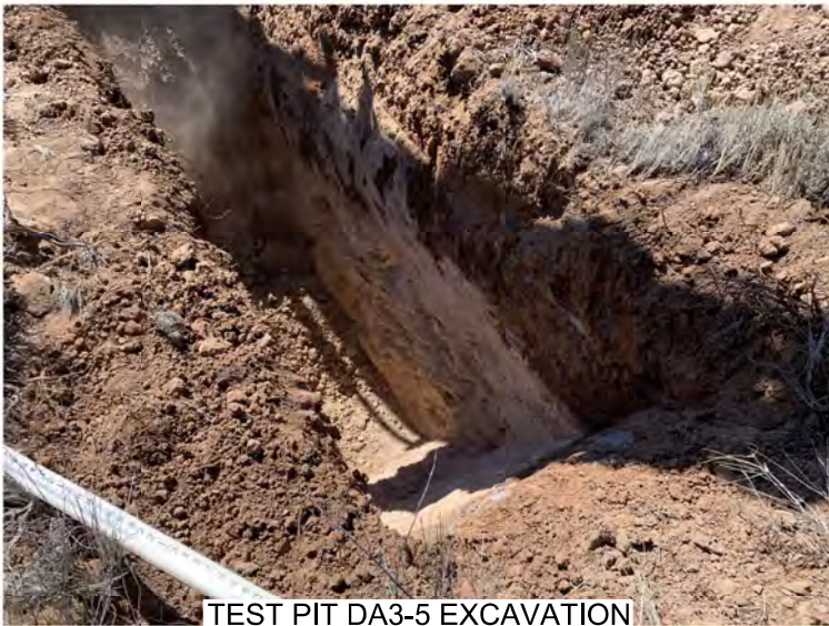
TEST PIT DA3-5 EXCAVATION
