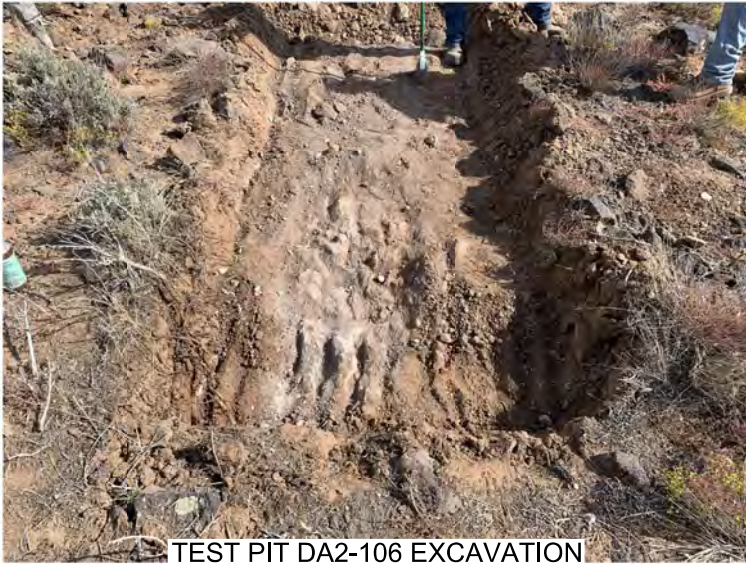
TEST PIT DA2-106 EXCAVATION
