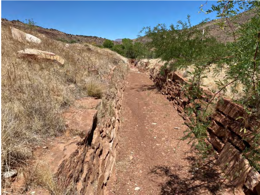
View of the improved section of Ditch 1 looking downstream (facing northwest)
