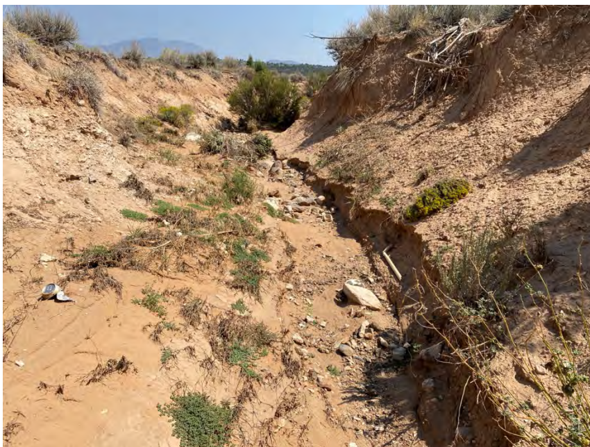
View of Wash 4 looking upstream where it exits the review area (facing east)
