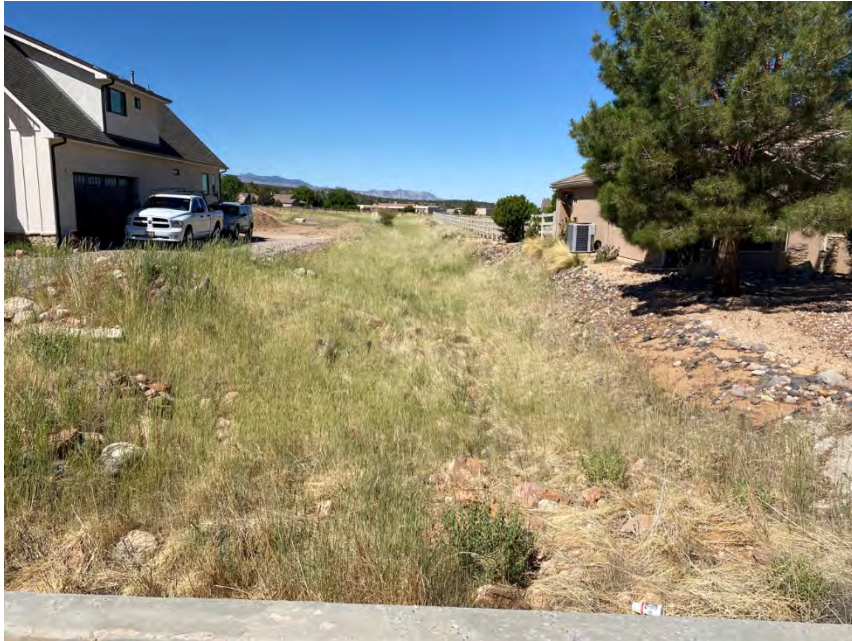
View of Wash 1 looking downstream from N Canyon Trails Dr. Note the barely distinguishable OHWM due to vegetation growth (facing southwest)
