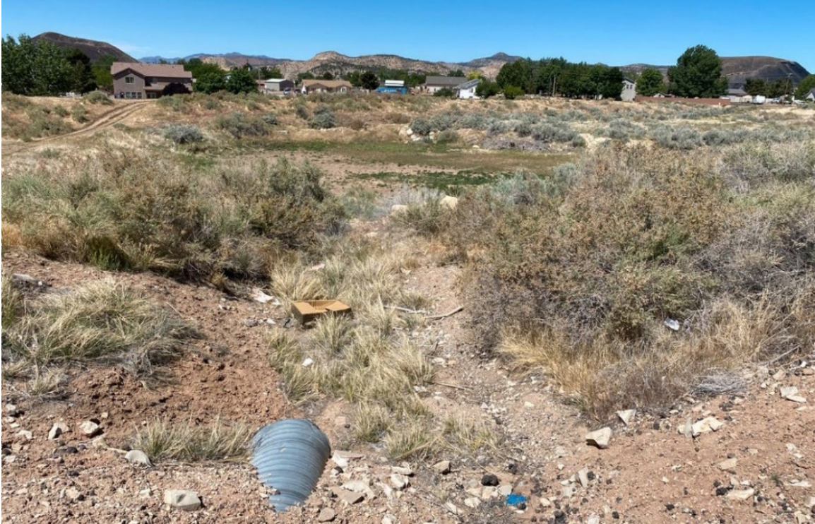
Photograph C-14. Existing Basin in Diamond Valley that would be repaired.
