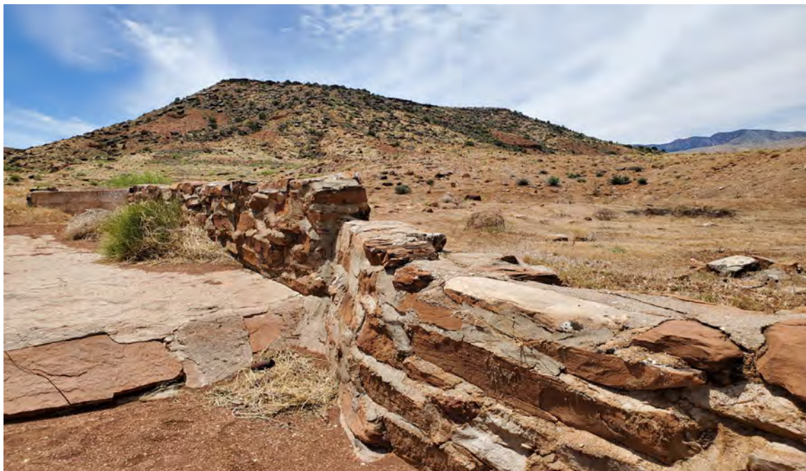
Figure 4. Overview showing a portion of site 42WS6523 historic flood control ditch in Shem Valley on Paiute (Shivwits) land. View to the northeast.
