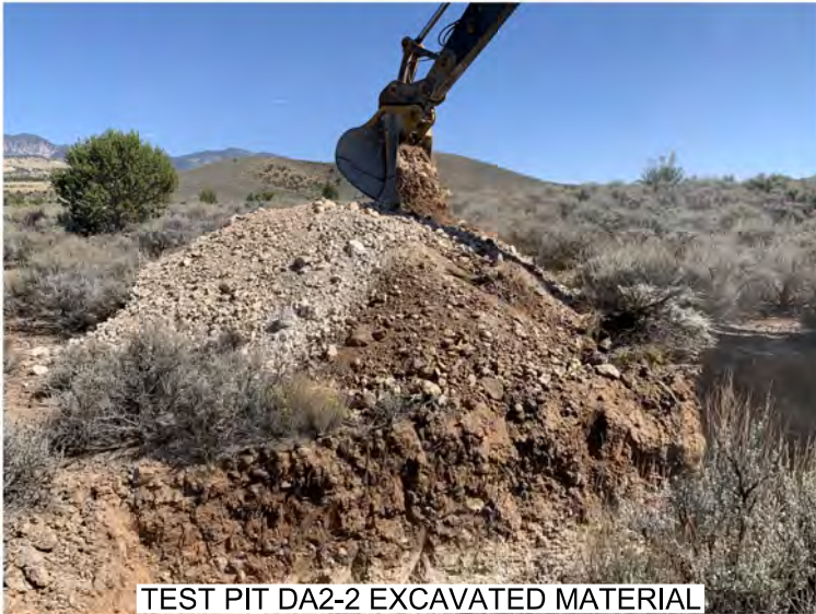
TEST PIT DA2-2 EXCAVATION
