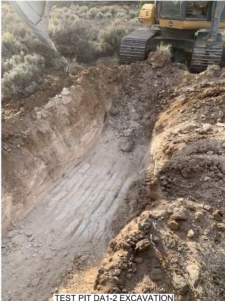
TEST PIT DA1-2 EXCAVATION
