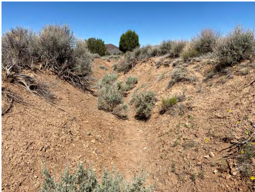
View of Wash 3 looking downstream where it enters the review area (facing northwest)
