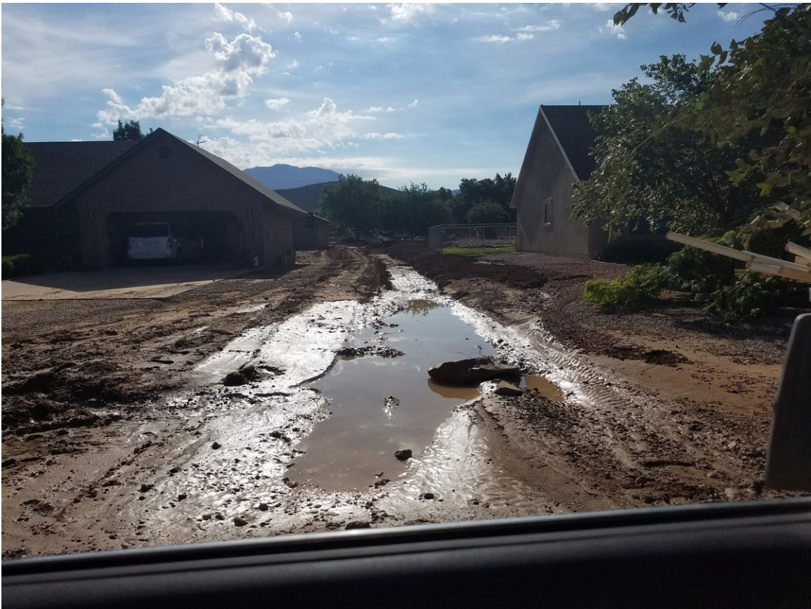
Photograph C-5. Flooding in Dammeron Valley, Utah.
