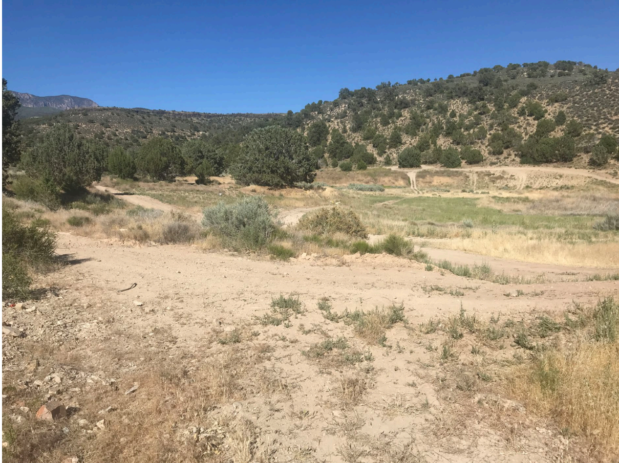
Figure 5-4. Existing Detention Basin in Diamond Valley to be Repaired
