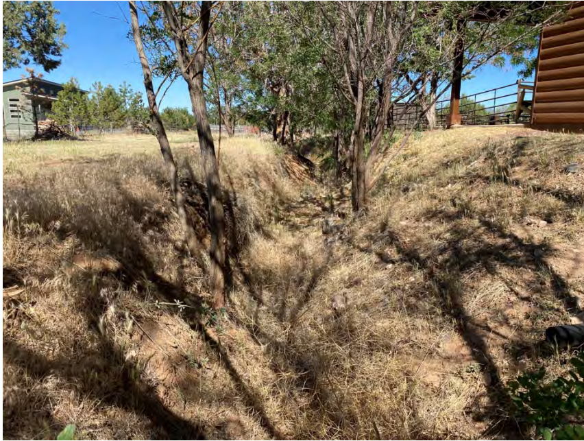
View of Wash 1 within the Vineyard looking downstream (facing west)
